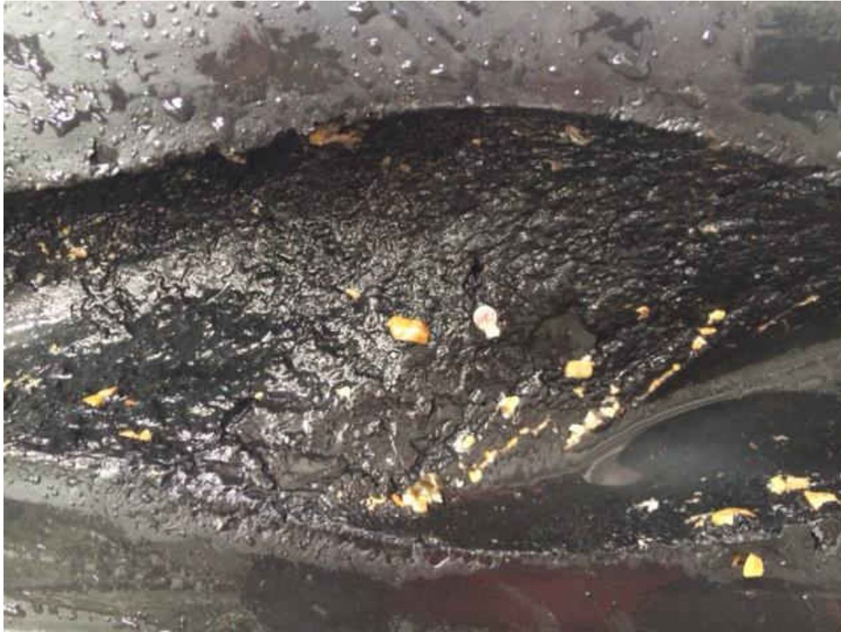
Damage to pump
