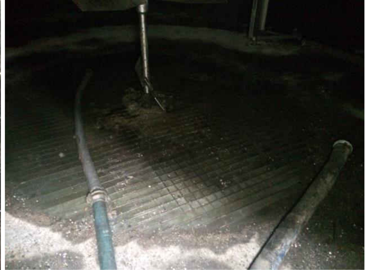
Scouring of tank
